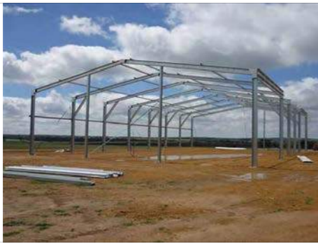
1. STEEL PORTAL FRAME
