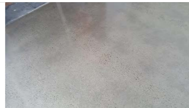
10. POLISHED CONCRETE SLAB WITH RANDOM AGGREGATE EXPOSURE
