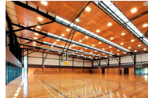
6. MARINE PLYWOOD CEILING LINING
